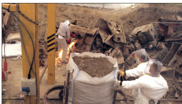
Clearing land contamination at Harwell
